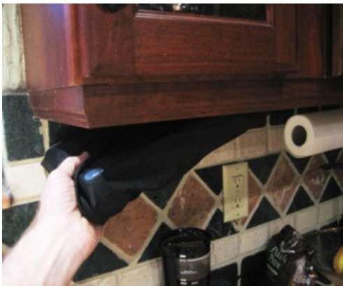
4. Use hot glue on mounting under cabinets, etc.
