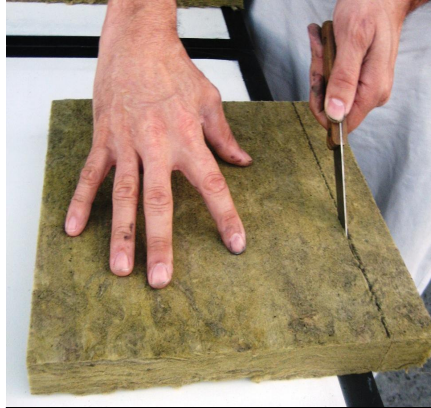
2. Use a serrated knife to cut QuietFiber material.
