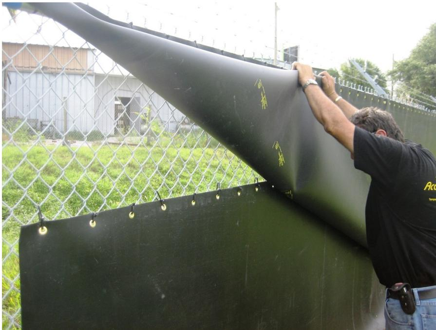
The Acoustifence is a unique 1/8th inch, 6' x 30' (3mm x 1.83m x 9.14m) heavy mineral filled, barium free viscoelastic acoustical material. It is made in the USA from all USA materials.
