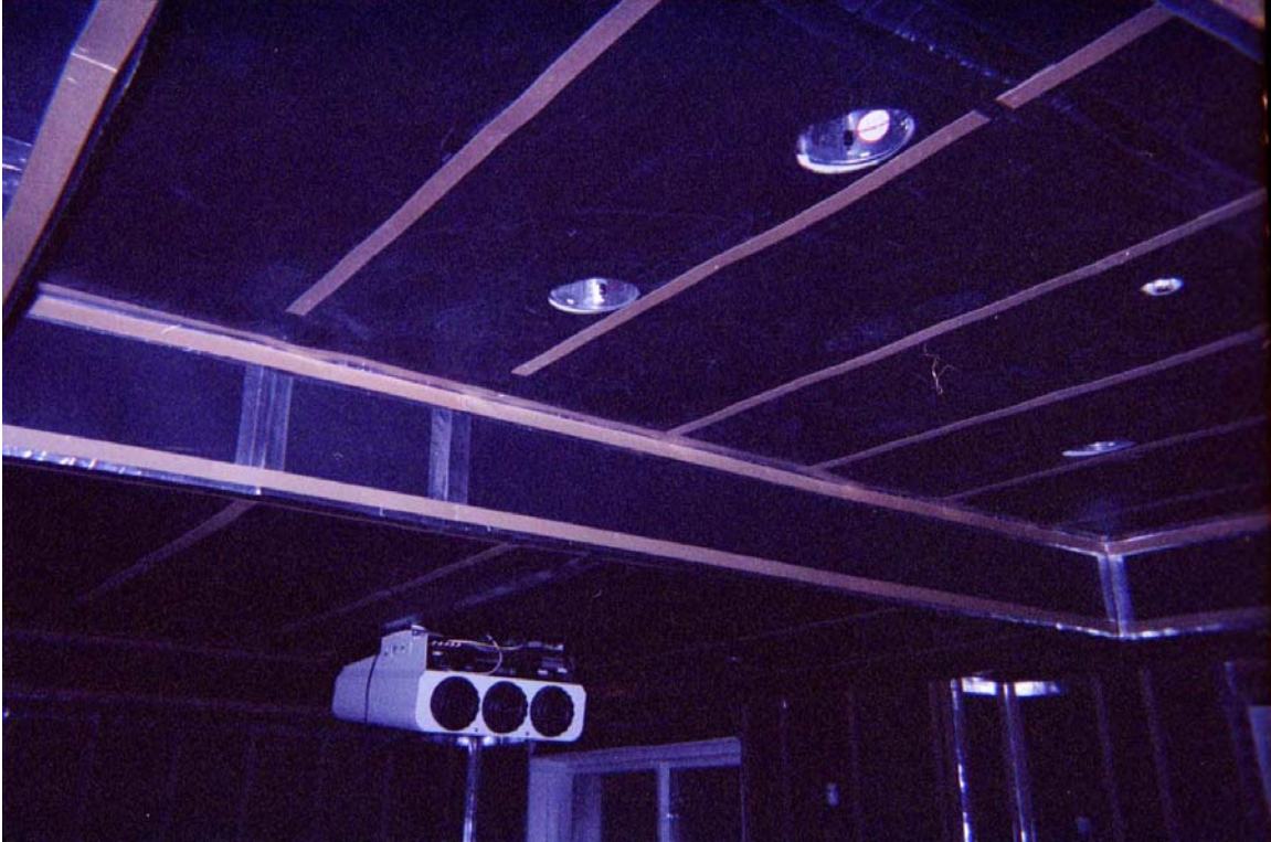
Photo 3 - finished ceiling showing can lights and soffit detail
